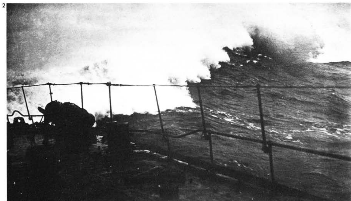
1 The Second Torpedo Boat Flotilla in battle formation. Note that the two lines ahead are staggered (Author's collection) 2 The wash of a B-Boat. Note the method by which the top half of the guard rails were cleared away for action (Bundesarchiv)
